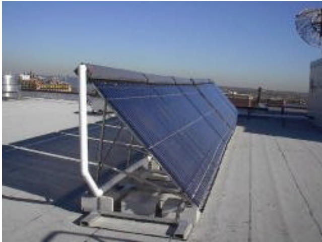
Figure 13: Installation costs are 14% of the total vacuum tube system costs.
