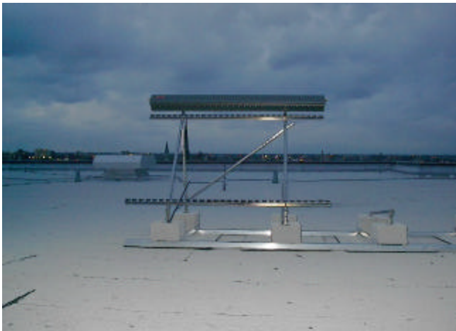
Figure 10: Manifolds are assembled at the job site using stainless steel hardware.
